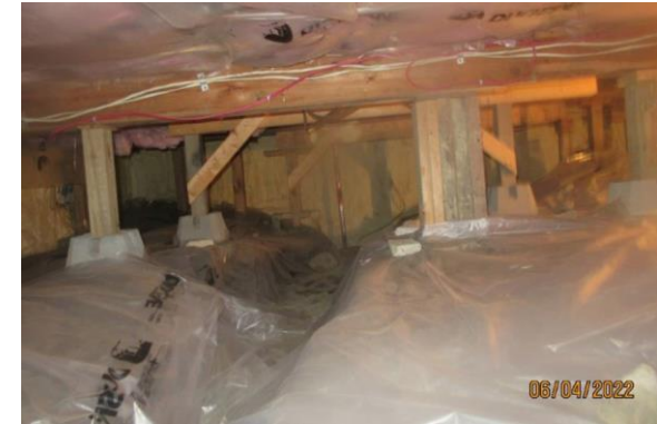
Renforcement artisanal de la structure
